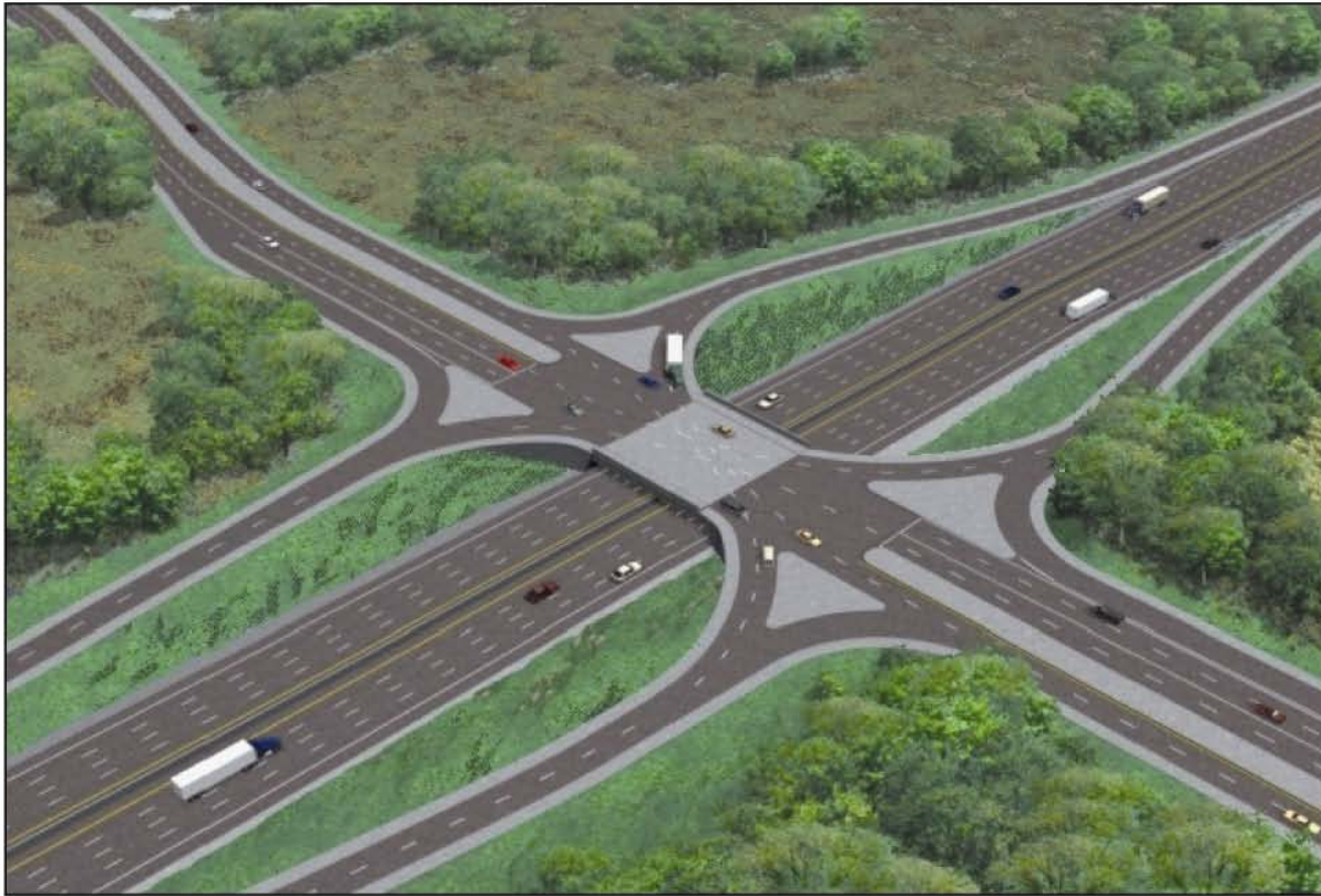
Figure 27 Single-Point Urban Interchange (SPUI)
