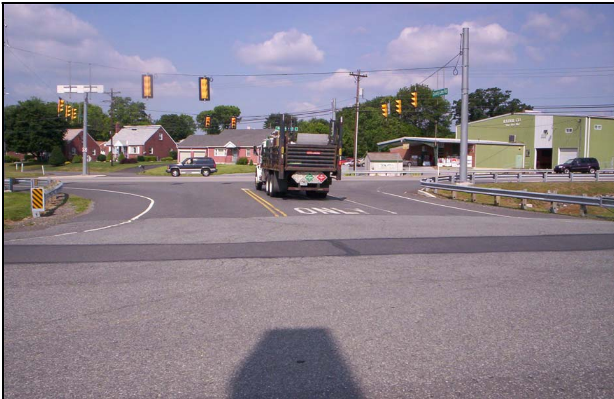
Pictured: Proximity of the Holly Road/County Line Road intersection to PA Route 100.
