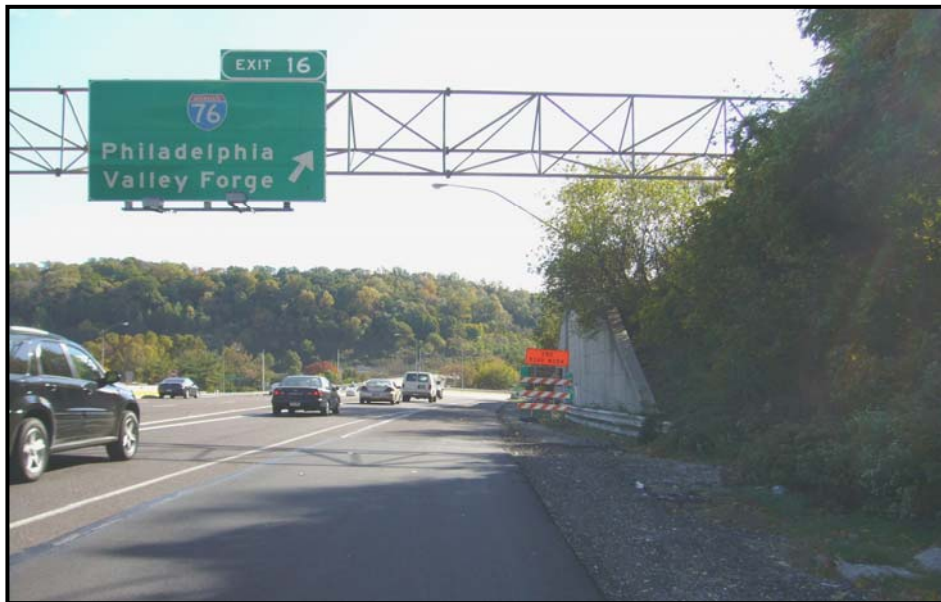
Figure 3: I-476 Southbound Exit Ramp
