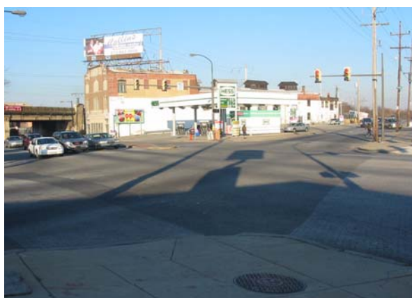
Inadequate road markings and poor access management (See location 24)
