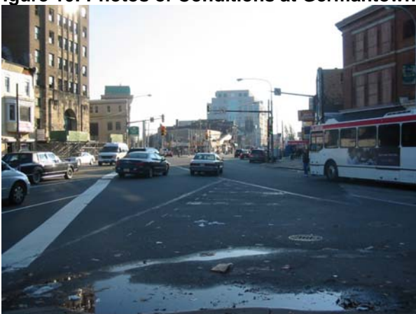
Inadequate lane markings and pedestrian facilities (See location 21)
