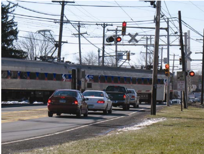
Above shows the at-grade train crossing at Bristol Road. Source: DVRPC, February 2008
