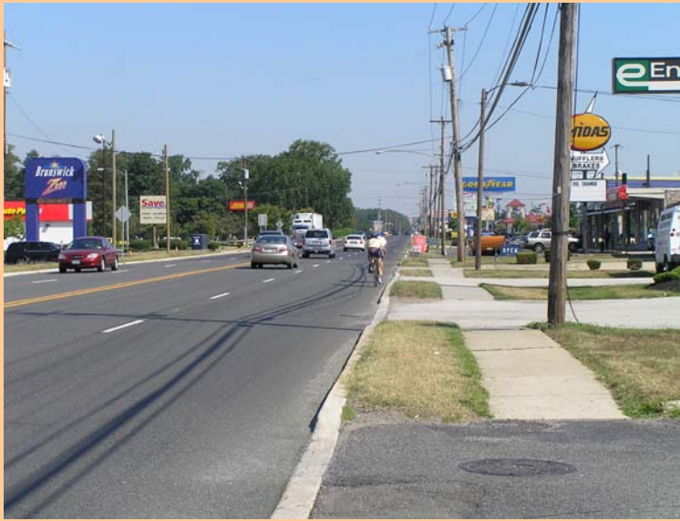
Existing NJ 47 configuration with bicyclists and motor vehicles sharing the same travel lane Source: DVRPC 2008
