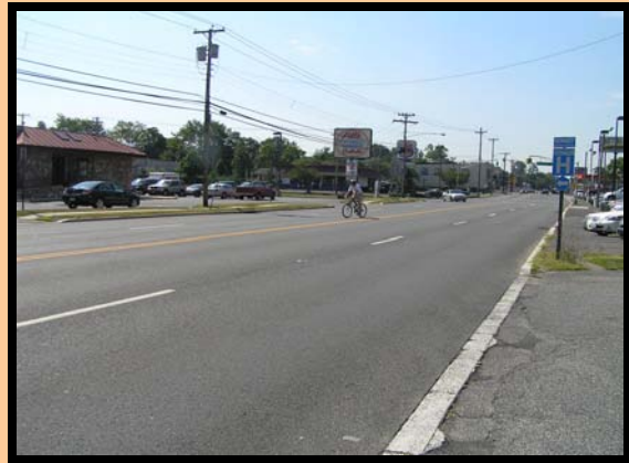
Land use in the study area is predominantly commercial. There are a large number of driveways on both sides of the roadway Source: DVRPC, 2008
