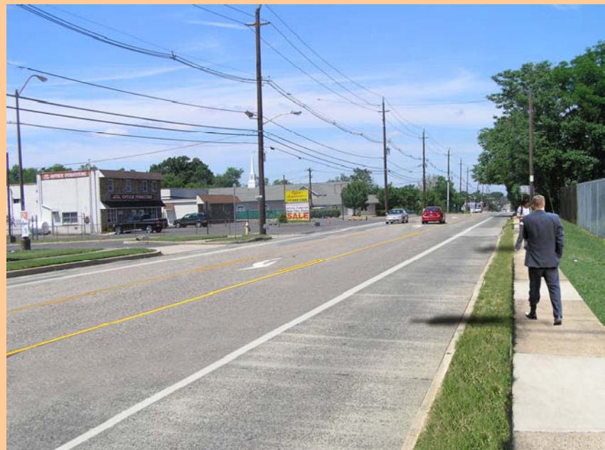
Rendering of the road diet conversion of Haddonfield Road with shoulder and sidewalk Source: DVRPC 2008
