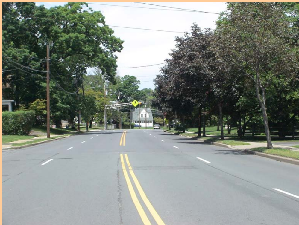
Existing Parkway Avenue configuration with pedestrian crossing Source: DVRPC 2008
