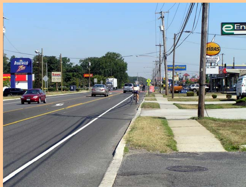
Rendering of the road diet conversion of NJ 47 with bicyclist using shoulder/bike lane Source: DVRPC 2008
