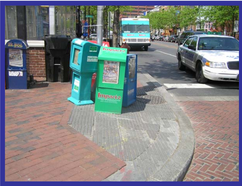
Newspaper boxes blocking the curb ramp at 2 nd Street
