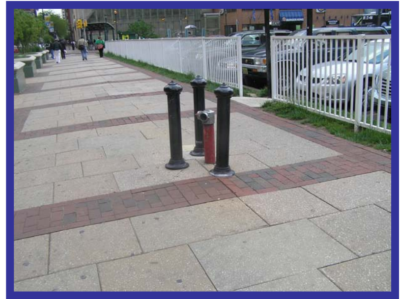
Standpipe in the middle of the sidewalk between 8 th and 9 th Streets
