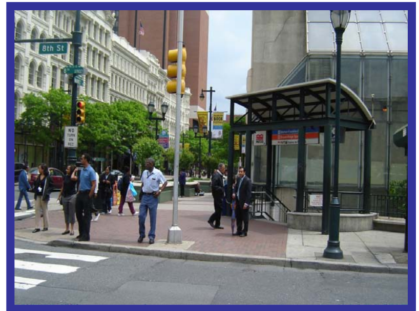
8 th Street Station for PATCO and the Broad Street and Frankfort Subway Lines
