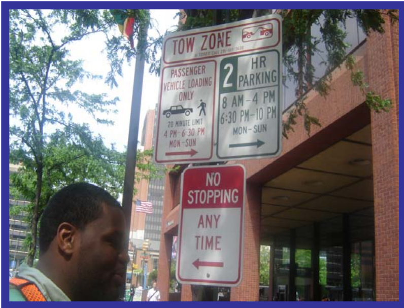
Signs mounted too low
