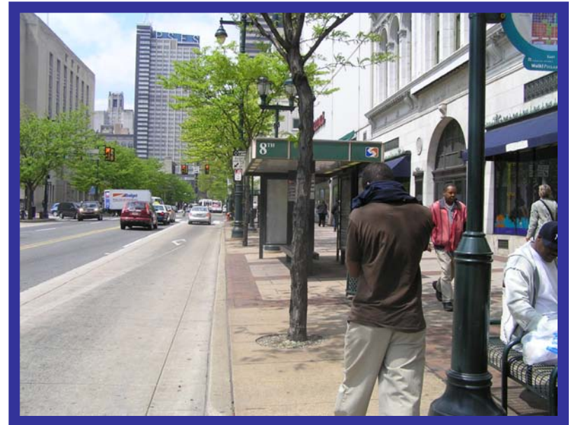
Bus lane pavement markings faded
