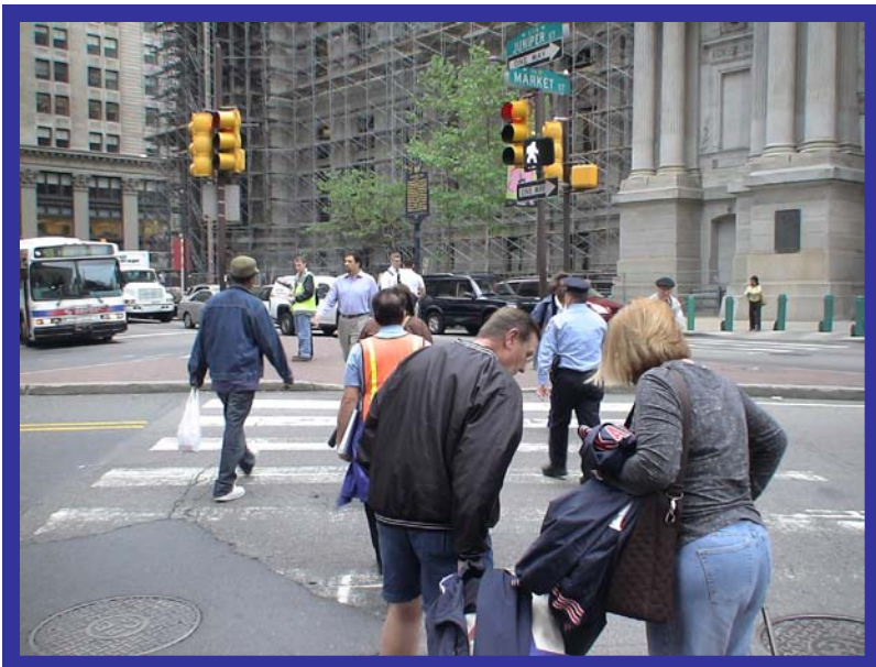
Faded crosswalk pavement marking at Juniper Street
