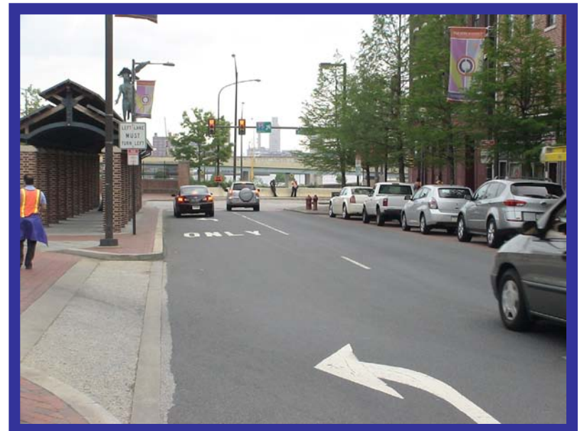
I-95 directional sign mounted on mast arm – no previous signage
