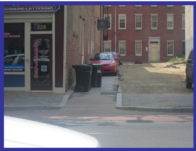
Crosswalk at South Bodine Street. Recommend raising the crosswalk to sidewalk level
