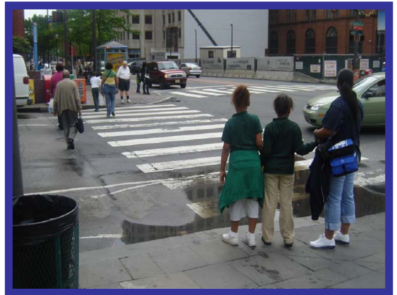
Pooling at the northwest corner of the 5 th Street intersection Pedestrian trying to cross 5 th Street
