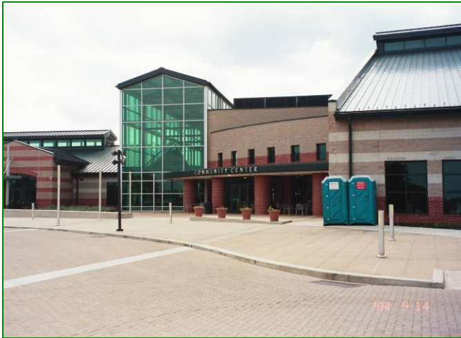
West Deptford Community Center Source: DVRPC, 2004
