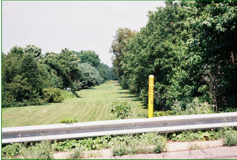
Pipeline right-of-way adjacent to Turnpike, Deptford Source: DVRPC, 2006
