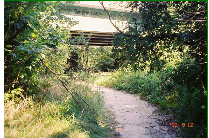
Unpaved trail under Route 55 along Chestnut Branch, Mantua Twp.
