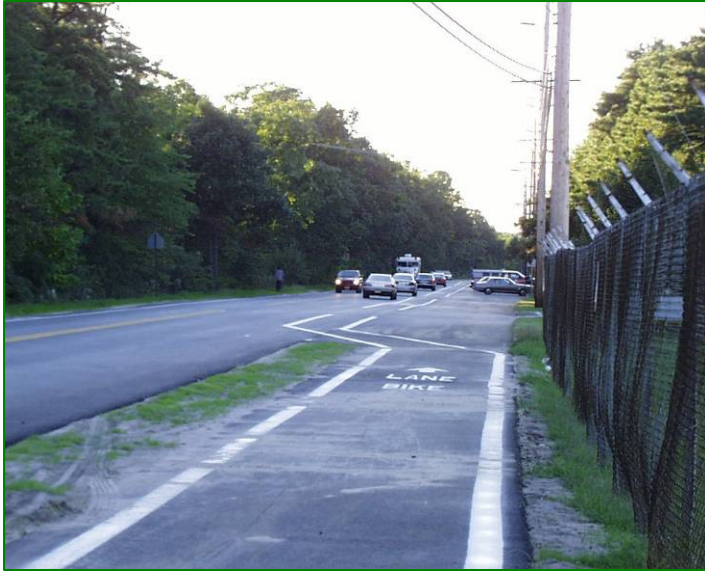
Improperly designed bikeway
