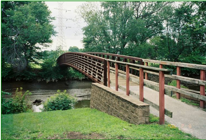
Judith E. Zaehring Bridge over Woodbury Creek, Woodbury
