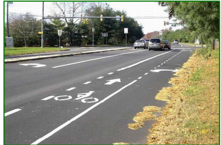
Acceptable designs for bike lane intersection approaches
