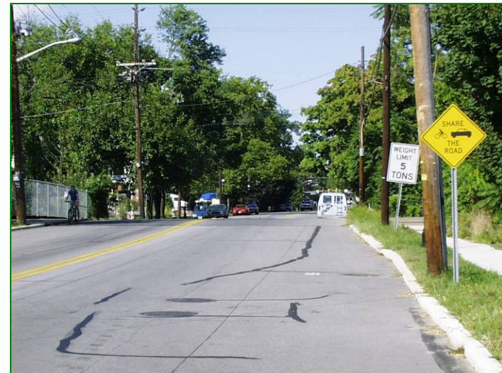
Shared roadway Source: DVRPC, 2001
