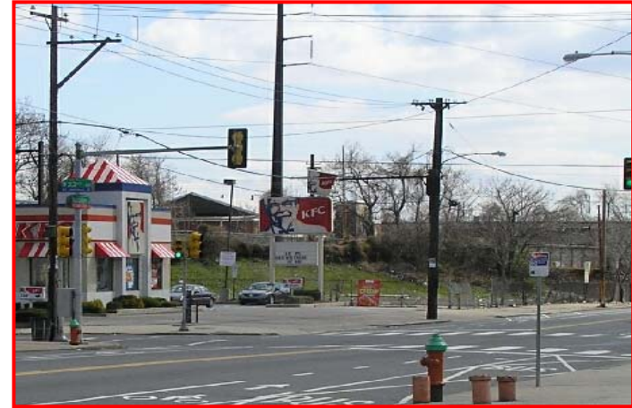
Driveways too close at intersection
