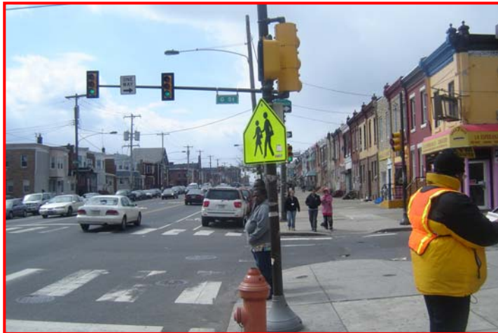
“School crossing” signs missing arrows or “Ahead”
