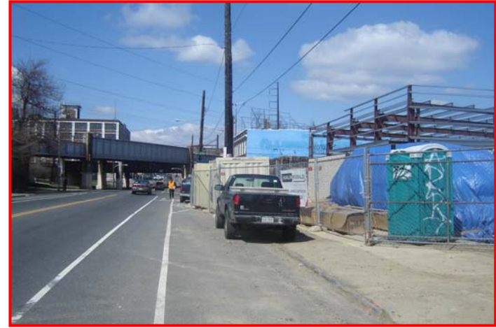
Construction blocks sidewalk
