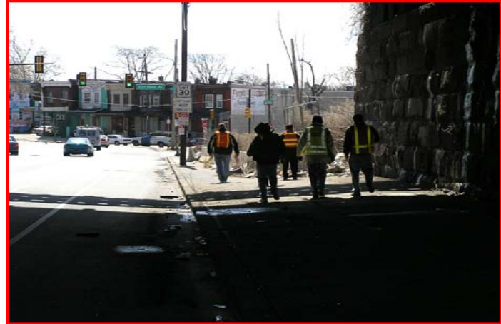
Inadequate lighting under bridge
