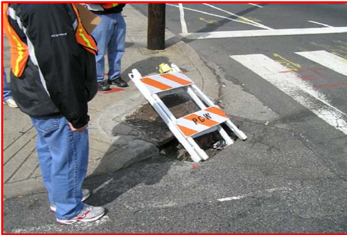
Drainage inlet grate located in the crosswalk
