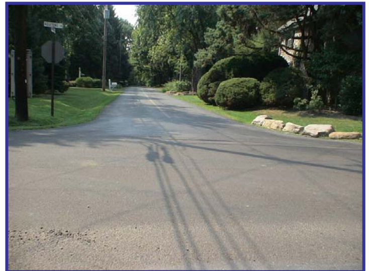
Rocks at corner of Aquetong and Old Windy Bush Roads in the clear zone
