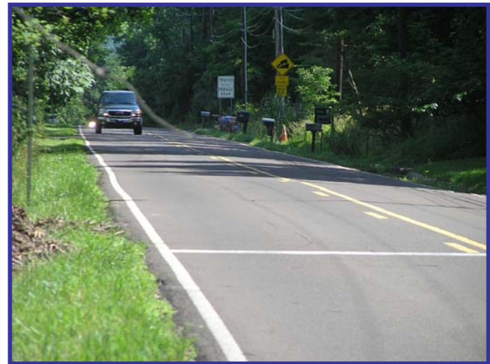
Windy Bush Road looking north at Cornwell Drive – passing zone, narrow shoulders
