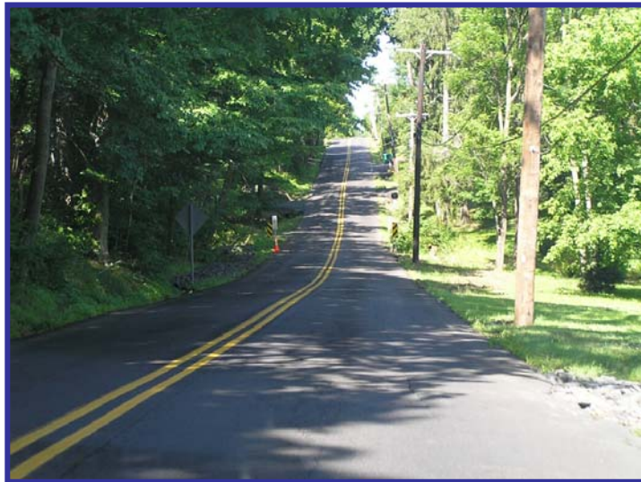
Utility poles in the clear zone on Aquetong Road east of Sugan Road
