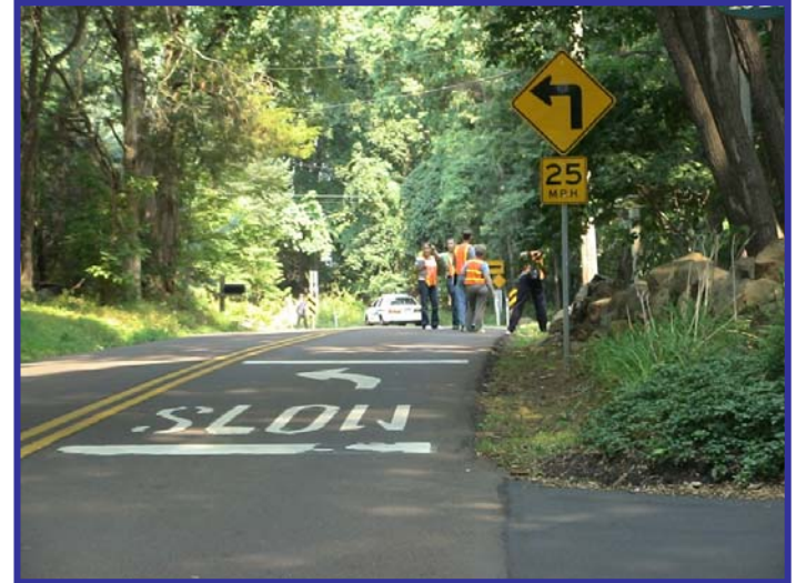
Deteriorating pavement marking on Aquetong Road
