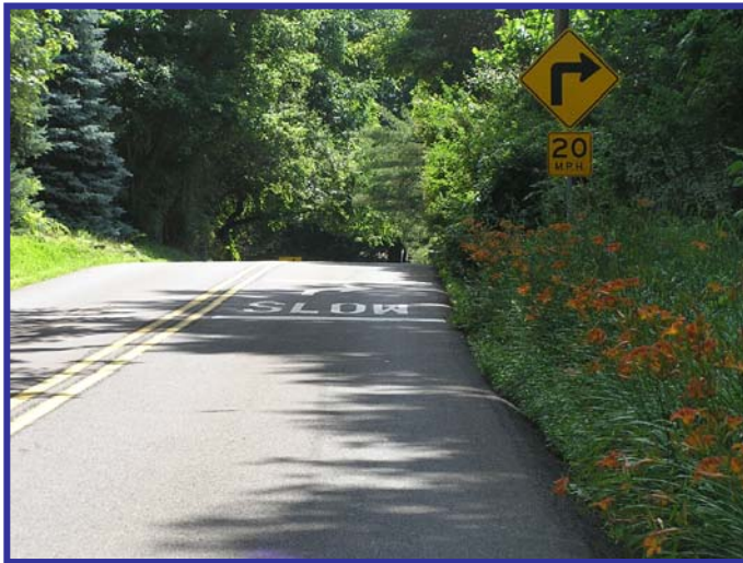
Pavement marking on Aquetong Road
