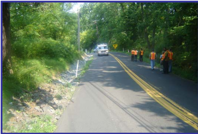
Deteriorating delineator pole on Aquetong Road east of Sugan Road
