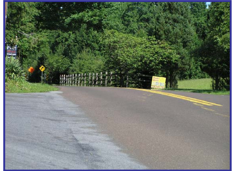
Vegetation at the intersection of Aquetong Road and Cover Bridge Road limits sight distance looking west
