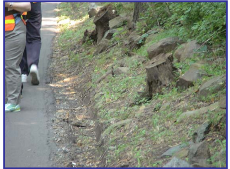
Rocks and tree stumps along Aquetong Road in the clear zone
