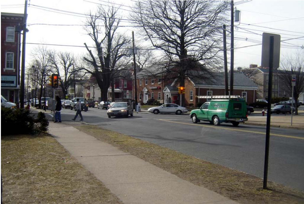
Hamilton Avenue and Chestnut Street intersection showing post-mounted signals
