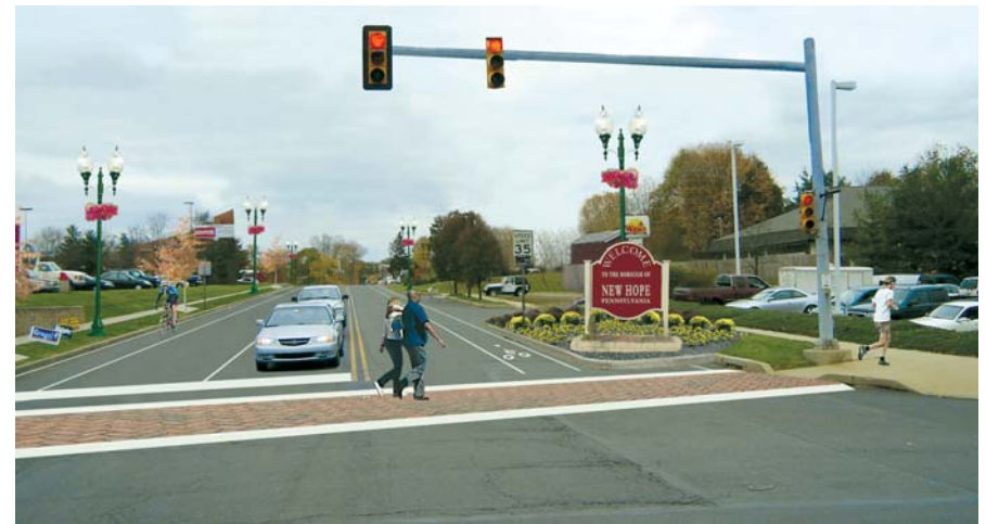
Figure 5: Gateway at Sugan Road and PA 179 - After
