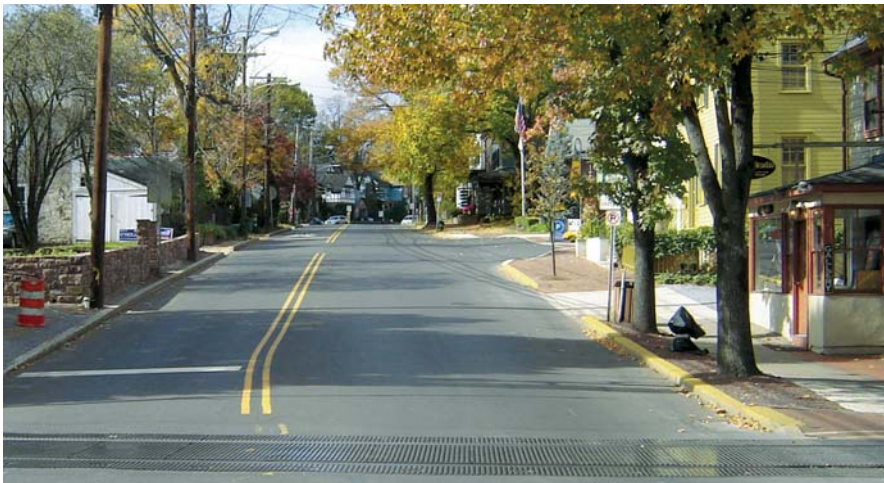
Figure 10: PA 179: Kiltie Drive to Ferry Street - Before
