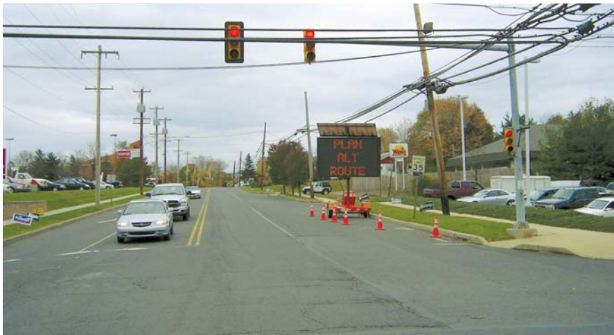
Figure 4: Gateway at Sugan Road and PA 179 - Before
