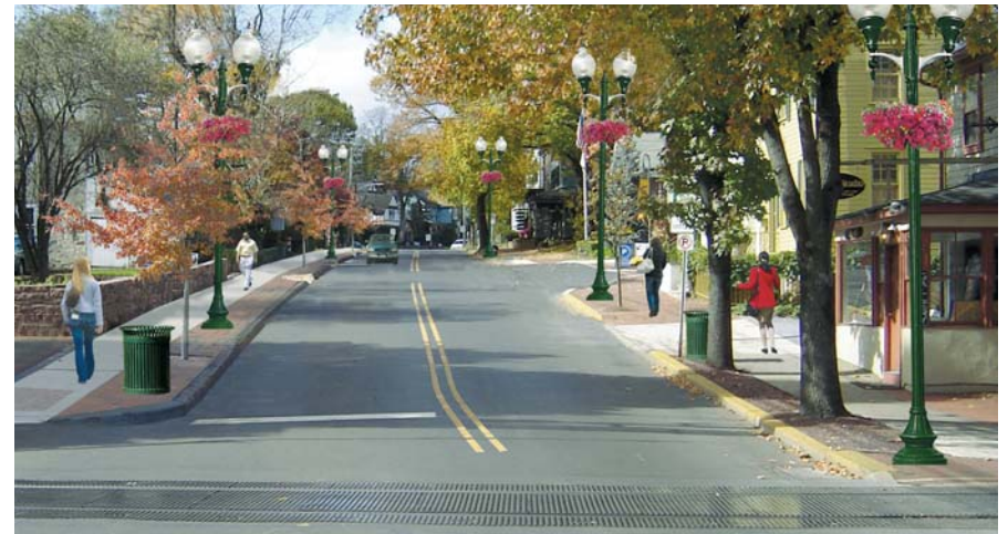
Figure 11: PA 179: Kiltie Drive to Ferry Street - After
