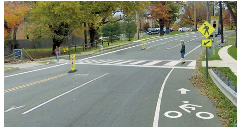
Figure 9: PA 179: Old York Road to Kiltie Drive - After
