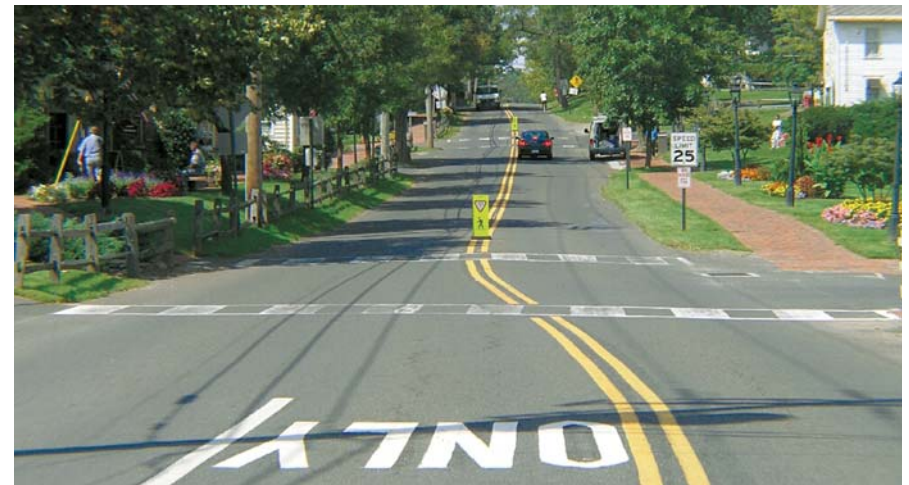
Figure 2: View of Street Road Crosswalks Adjacent to Southbound Left-Turn Lane
