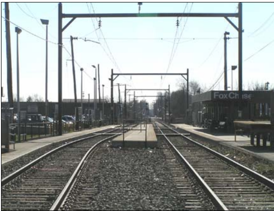
Both platforms of the Fox Chase Station from the terminus at Rhawn Street.
