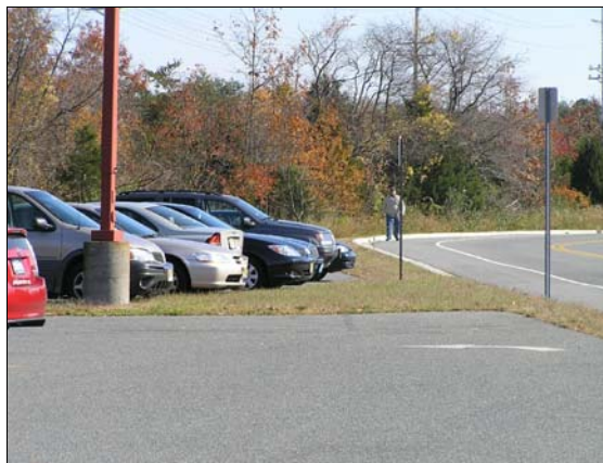
A pedestrian approaches Atco Station along C.W. Haines Boulevard. A lack of sidewalks throughout the study area hinders access by pedestrians.
