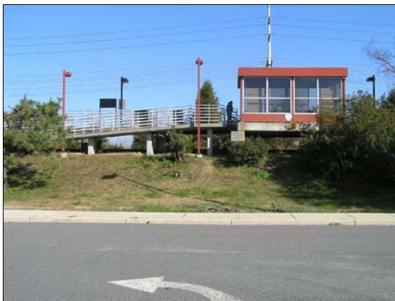
Atco station viewed from the parking lot south of the platform.
