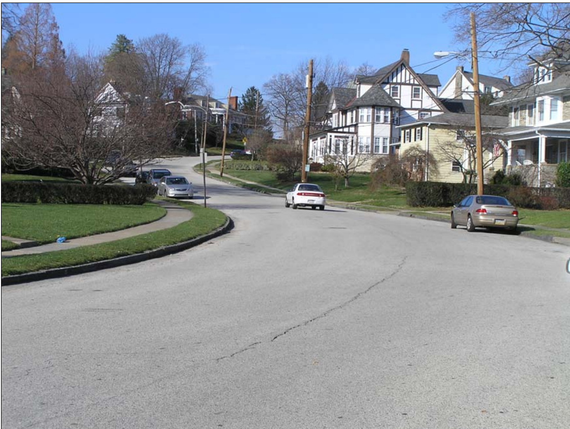
Roberts Avenue from Geneva Avenue to Mt. Carmel Avenue, north of Glenside station. Factors yielding the highest possible BLOS score include low traffic intensities (an estimated AADT of 1,250 and 25-mph speed limit) and a relatively wide cartway width (34 feet).
