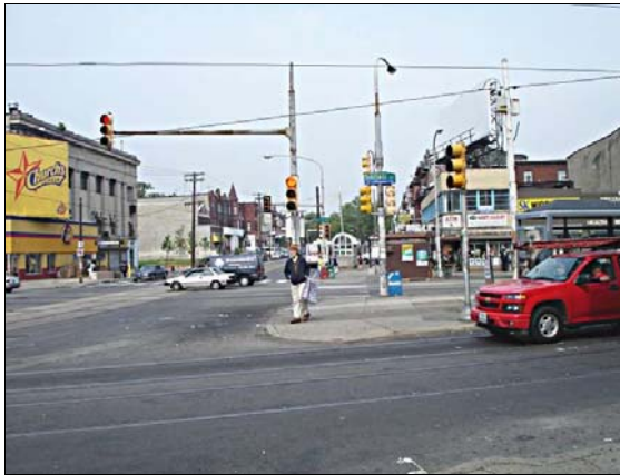
Broad/Erie/Germantown intersection viewed from northeast corner of Germantown Ave. and Erie Ave. (Broad Street runs left to right in background). Photo courtesy Orth-Rodgers & Associates.
