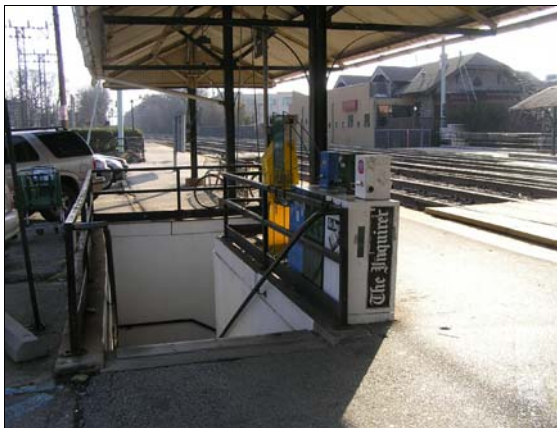
An underground passageway allows transfer between both sides of the station.
