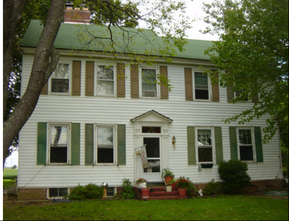
26. 132 Halltown Road Benjamin Wright House. About 1770 Benjamin and Ruth Wright came from Chesterfield in Burlington County to build this exceptionally fine Georgian frame house. Most of its interior architectural details including corner fireplaces with chip-carved mantels, chair rails, and original stairways have been preserved. 2 Exterior now covered with aluminum siding.
