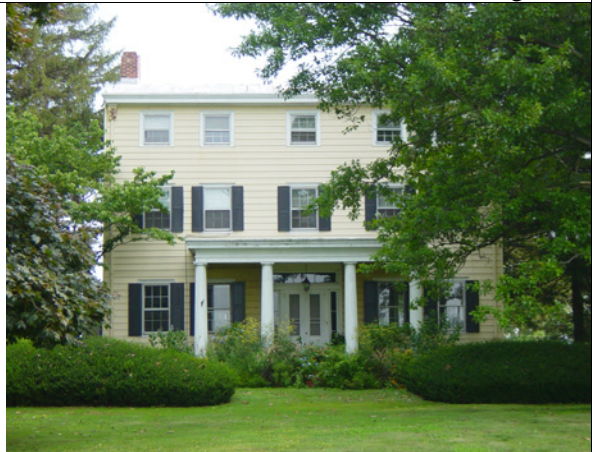
28. 84 Nimrod Road Sarah Bassett Griscom House. Frame Greek Revival house built by Benjamin Bassett for his daughter Sarah and her husband Barclay Griscom about 1854. The original house did not have fireplaces because it was designed to be heated with Franklin stoves. 2 Exterior now covered with aluminum siding.
