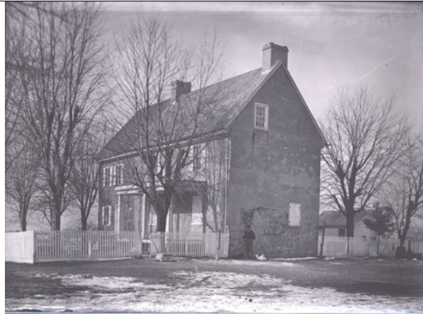
48. 466 Quaker Neck Road Hypolyte LeFevre House. This important brick house was built by Hypolyte LeFevre, Jr in the very early 18 th century. A brick with the date 1707 was found, which may indicate the year of construction. 2 The historic photo by Thomas Yorke 8 shows how the house looked in 1887. The left side appears to have been built after the right, but still sometime in the early 18 th century. The house has survived a disastrous fire and is quite altered today. Hypolyte LeFevre Sr., a French Huguenot escaping religious persecution in France, migrated to Fenwick's colony and purchased 6000 acres along with John Pledger. He died in 1698, and his son subsequently built this house on his inherited 3000 acre plantation. 2
