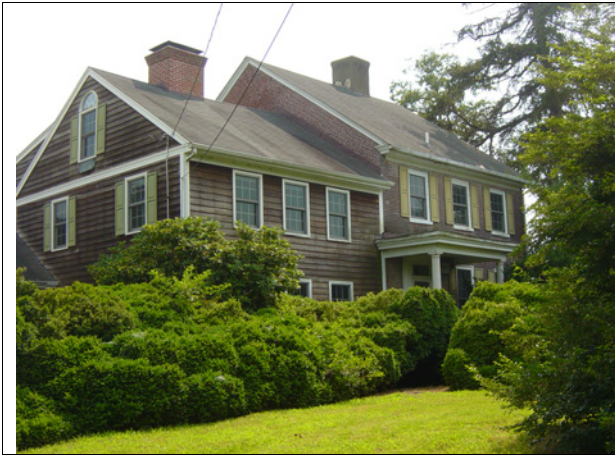
45. 663 Quaker Neck Road Brick section may have been built in the last quarter of the 18 th century. The porch is a later addition. The frame section is dated 1811. The frame section was re-sided in the 1990's. The interior of both sides has been altered.
