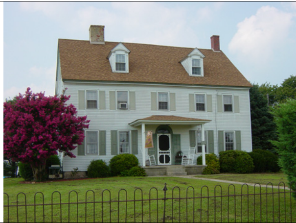
46. 606 Quaker Neck Road House appears to have been built in early 19 th century. The house has been covered with vinyl siding, and the porch has been added.
