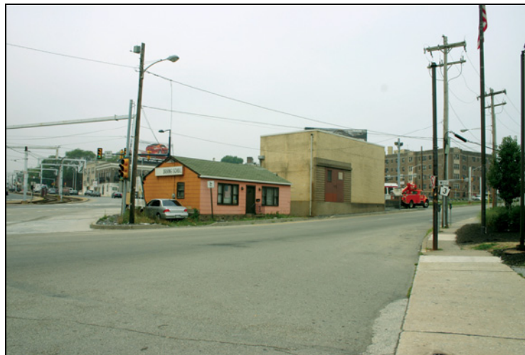
Buildings and catenary support located in West Chester Pike median at Garrett Road
