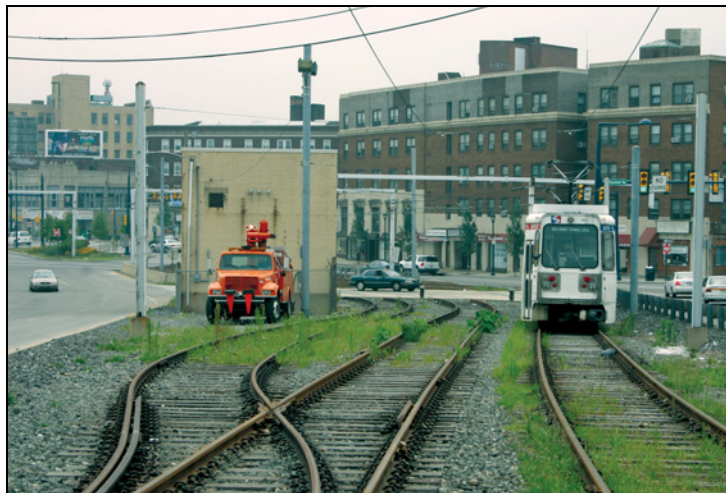
SEPTA spur line in median at Garrett Road
