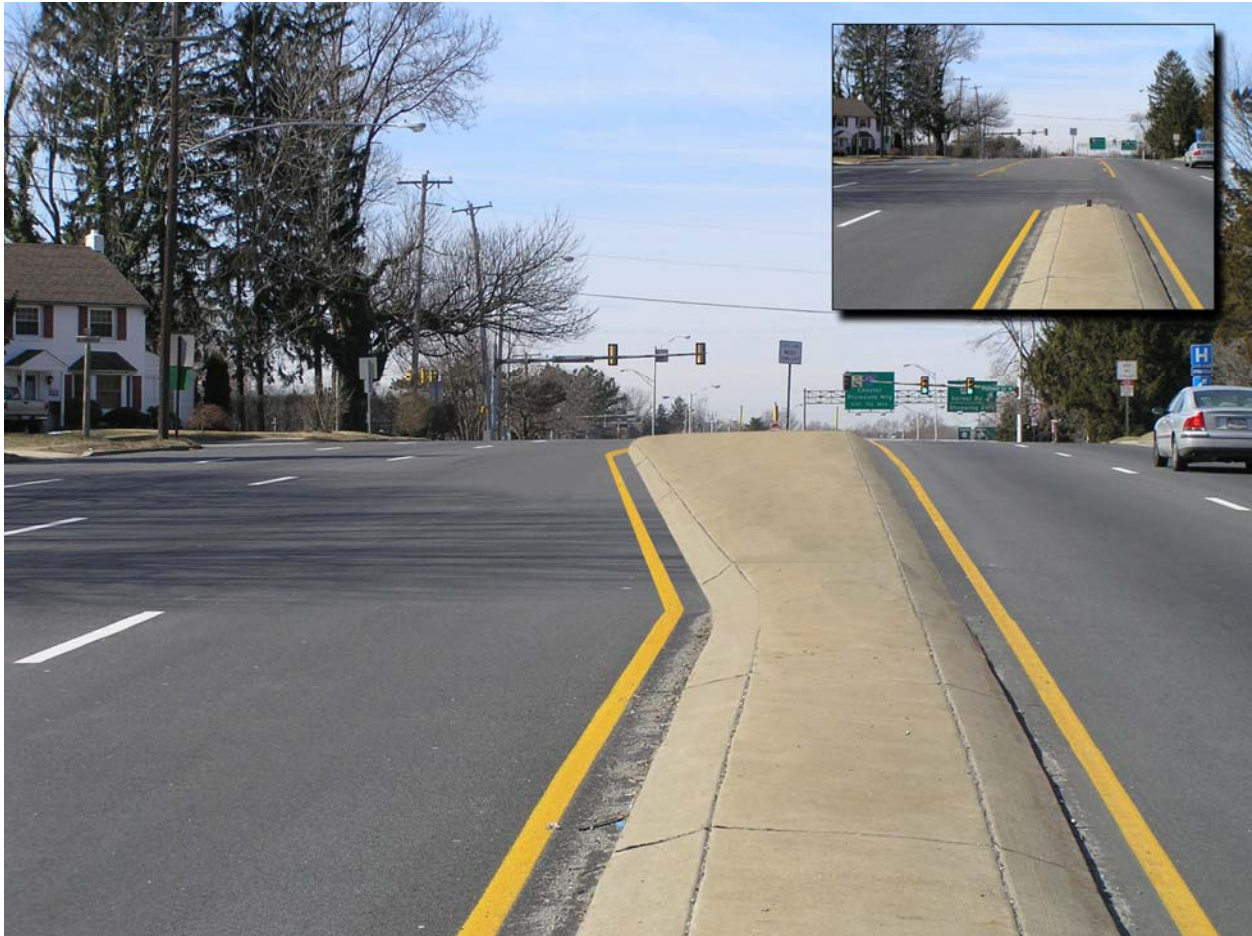
US 1 looking SB at Buttonwood Drive proposed median closure (inset: existing condition)
