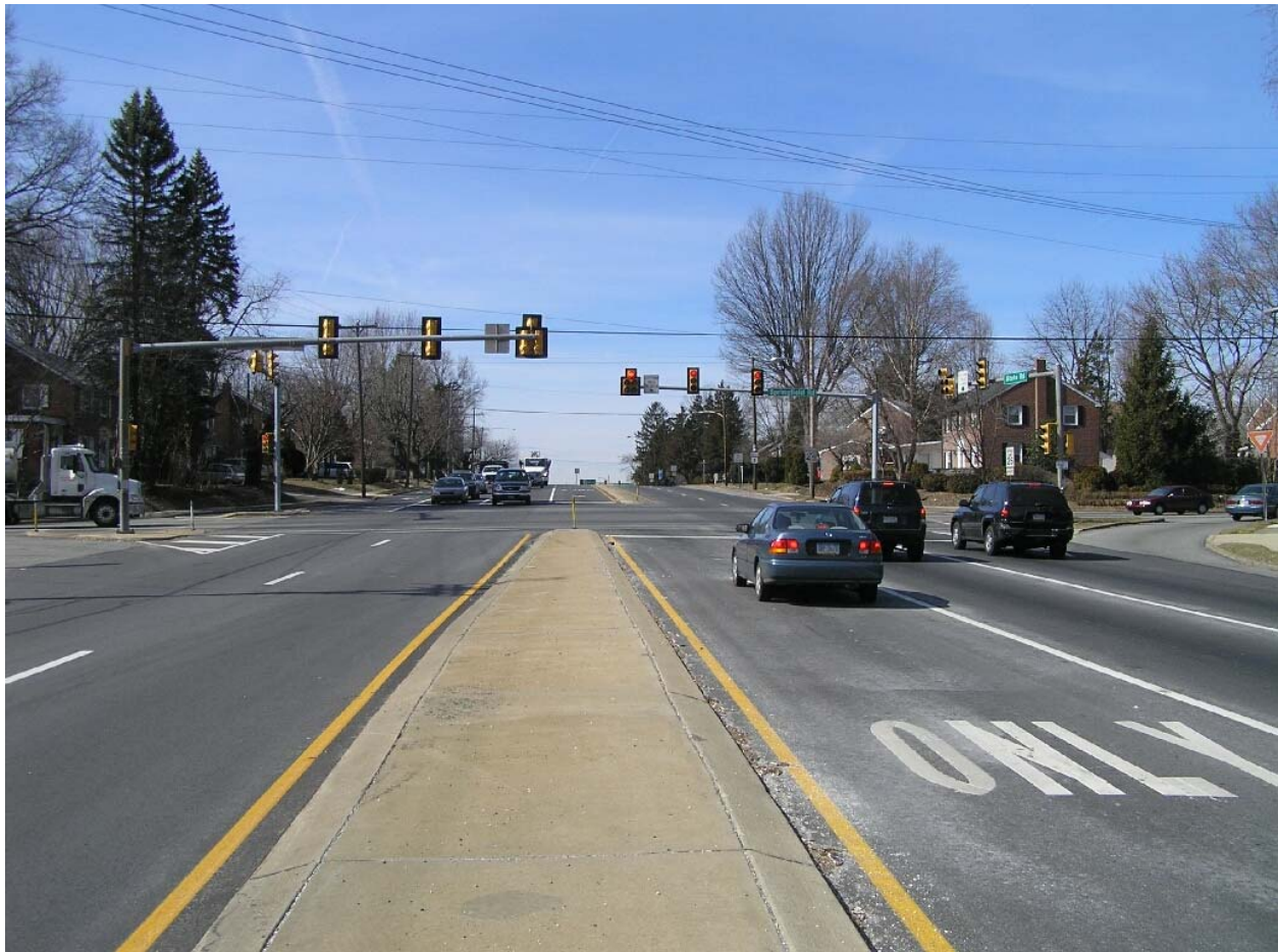
US 1 looking SB at Springfield Road
