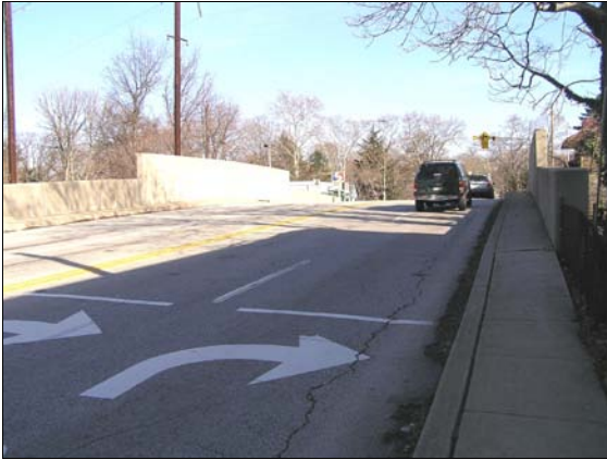
Montgomery Avenue bridge over rail tracks.
