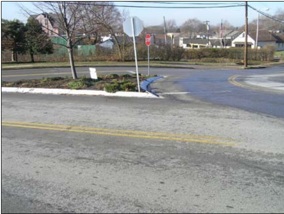
Lack of crosswalks at intersection of Bridge Avenue, Bruce Road, and Eherenport Avenue.
