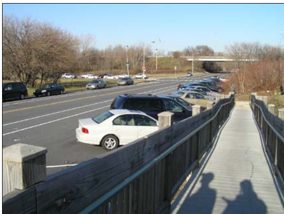
Diagonal parking along Mario Lanza Blvd. adjacent to station
