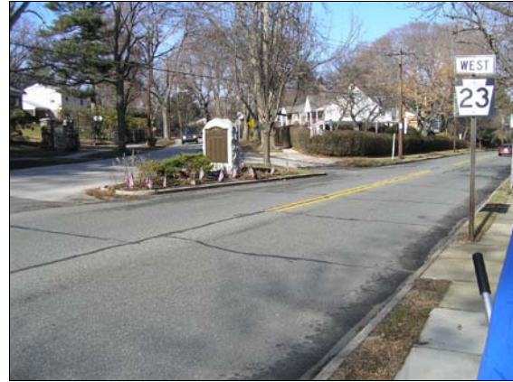
Lack of shoulder along Route 23 in the station area.
