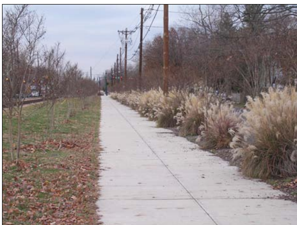
Buffered station access walkway along S. Broad St. (from Thomas Ave. to station platform) – vehicular cartway is to the right, rail line to the left
