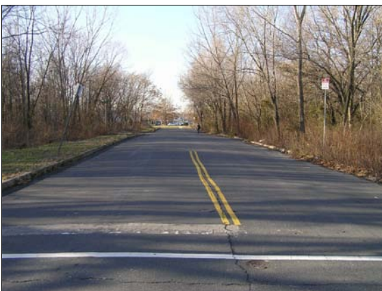
85 th street between Suffolk Place (background) and Eastwick Place.
