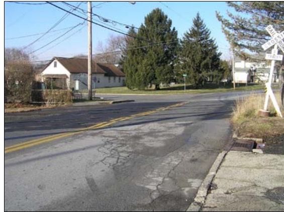
Lack of sidewalks adjacent to rail crossing (Eherenport Avenue).
