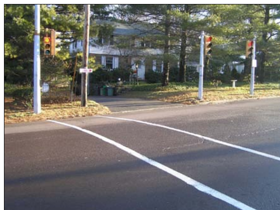
A crosswalk permits safe walking across Pennsylvania Avenue, but connects to no sidewalks on the northern side.
