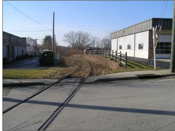
Abandoned rail line (viewed from Bruce Road / station parking area).
