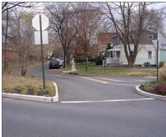
Problematic pedestrian access along Lippincott Avenue south of Broad Street (viewed from platform area)
