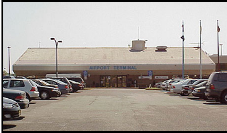
Trenton Mercer Airport Terminal
