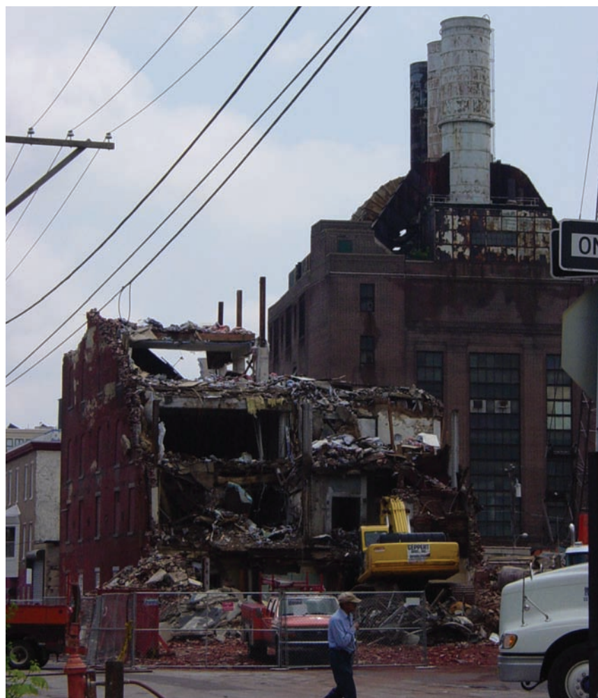
Demolition of historic loft structure
