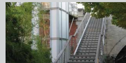
The viaduct becomes an elevated pedestrian walkway with garden spaces and access to the street at almost every block.
