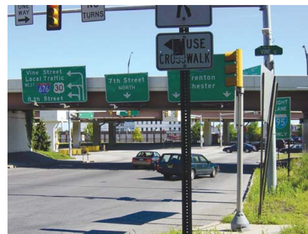
Vine Street Underpass at 7th Street - blank underpass walls and wide turning radii make for an unfriendly pedestrian environment.
