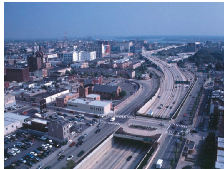
The Vine Street Expressway cuts a wide swath through Chinatown
