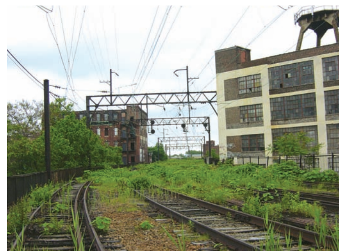
The Reading Railroad Viaduct
