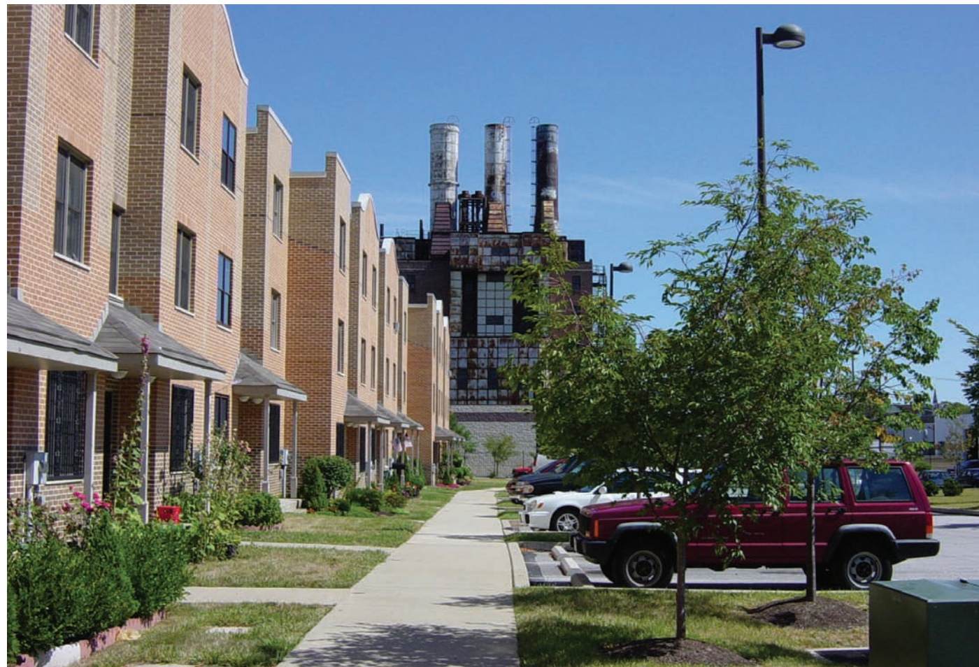
Tri-Gen co-generation plant and Hing Wah Yuen housing
