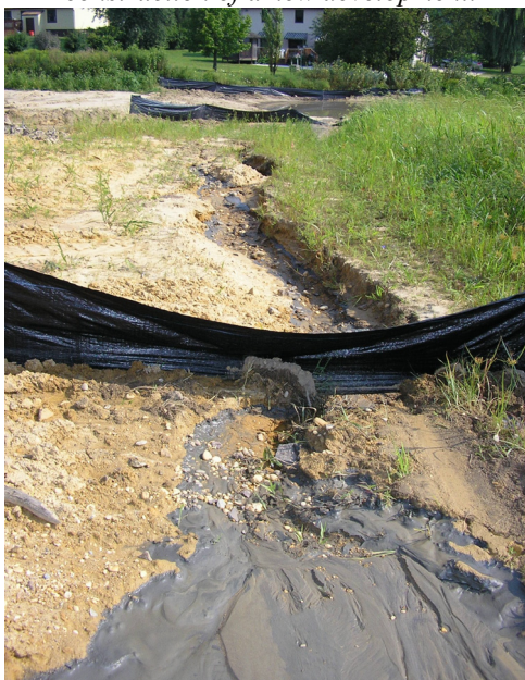
Source: Gloucester County Soil Conservation District
