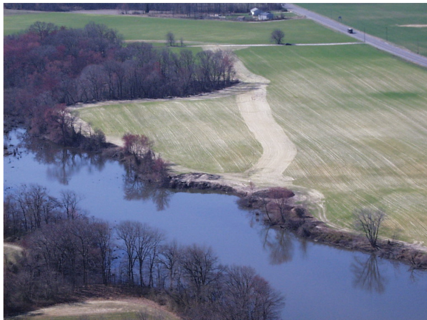
Example of an inadequate buffer and of streambank erosion
