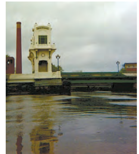
The Federal Street Bridge, courtesy of Fred Stine
