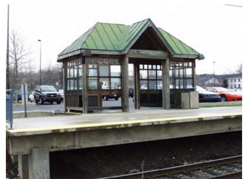
Station platform and shelter
