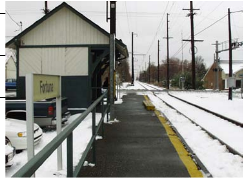
Station platform and shelter
