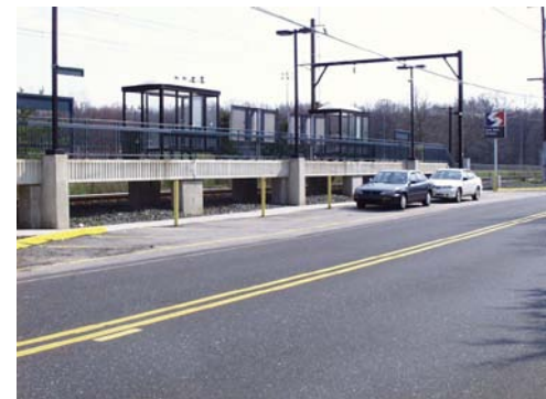
Station platform, shelters, and passenger drop-off area
