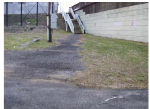
Inbound stairway and walkway
