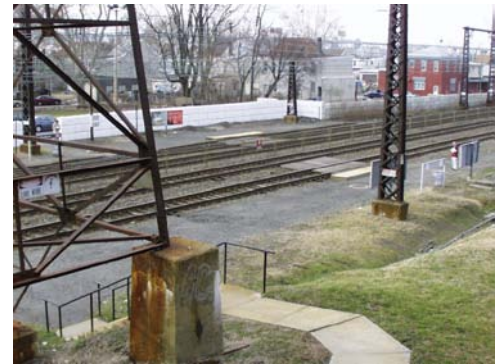
View of station from outbound stairway
