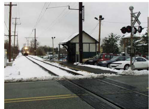
View of Cowpath Rd. grade crossing (foreground) as inbound train approaches
