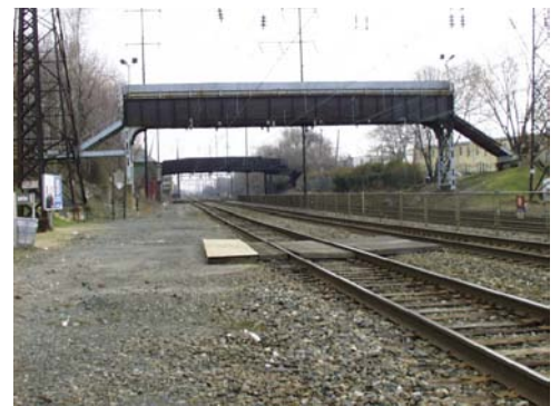
Outbound platform and walkway for crossing tracks
