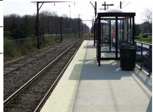
Station platform and shelters
