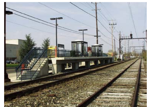
Station platform, shelters, and amenities
