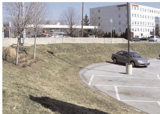
Above: The concrete barrier at the southeast corner of Butler Pike and Ridge Pike prohibits pedestrians. Shoppers must go around the barrier. (March 2001)
