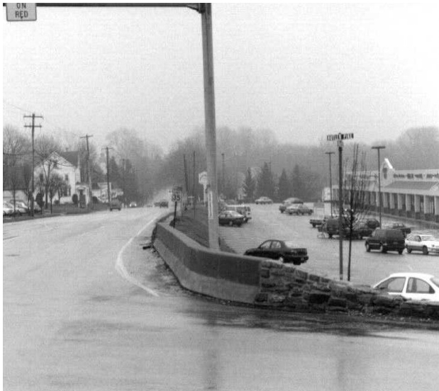
Above: Southeast corner of Ridge and Butler Pike, a wall prohibits safe access to shopping center for pedestrians. (November 2000)
