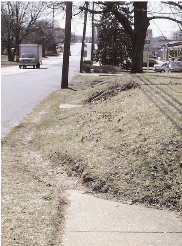
Above: Worn dirt and gravel paths indicate a desire for sidewalks. (March 2001)
