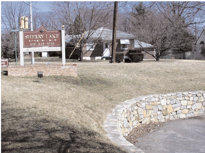
Left: The steep embankment on the southeast corner of the Butler Pike and Keys Street/ Cedar Grove Road, prohibits pedestrians of Sherry Lake Apartments. Pedestrians must go around the barrier. (March 2001)
