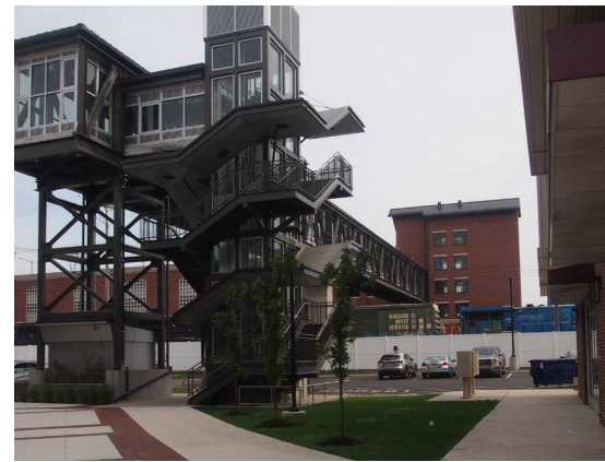
Pedestrian bridge connection to SEPTA parking garage and train station
