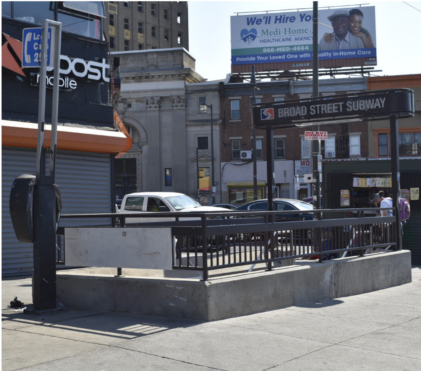
EXISTING ERIE STATION ENTRANCE
