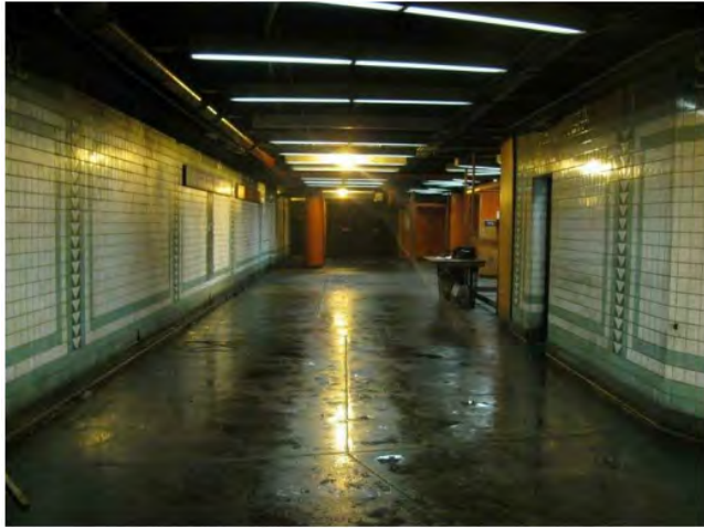
EXISTING CONCOURSE LOOKING SOUTH
