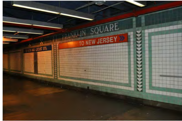
EXISTING CONCOURSE TILING
