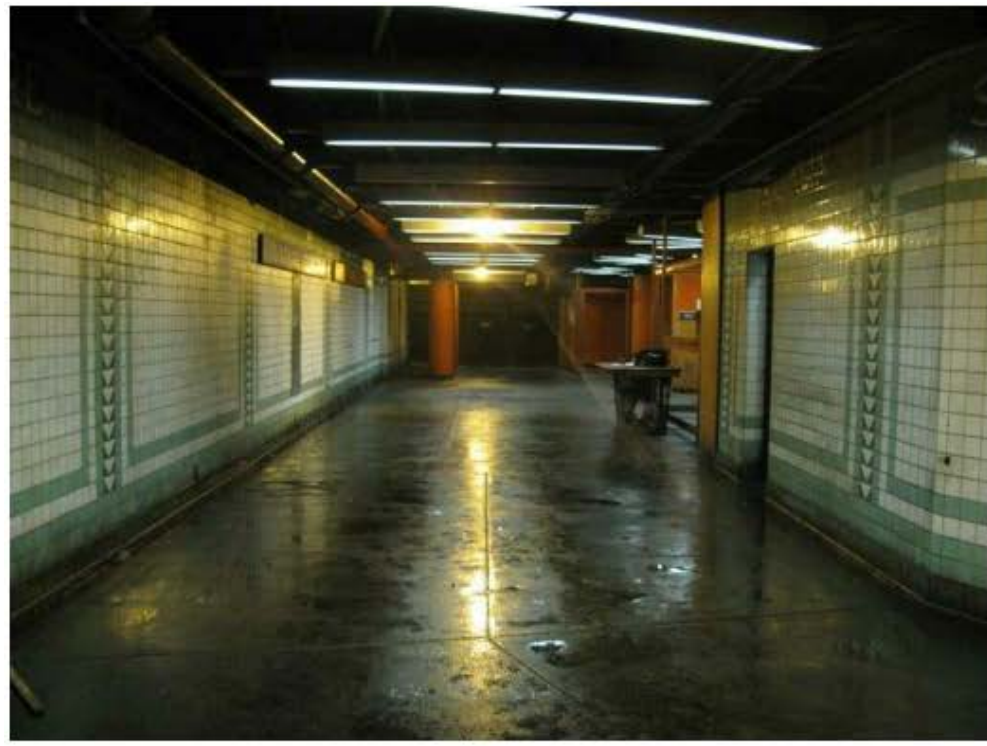
EXISTING CONCOURSE LOOKING SOUTH
