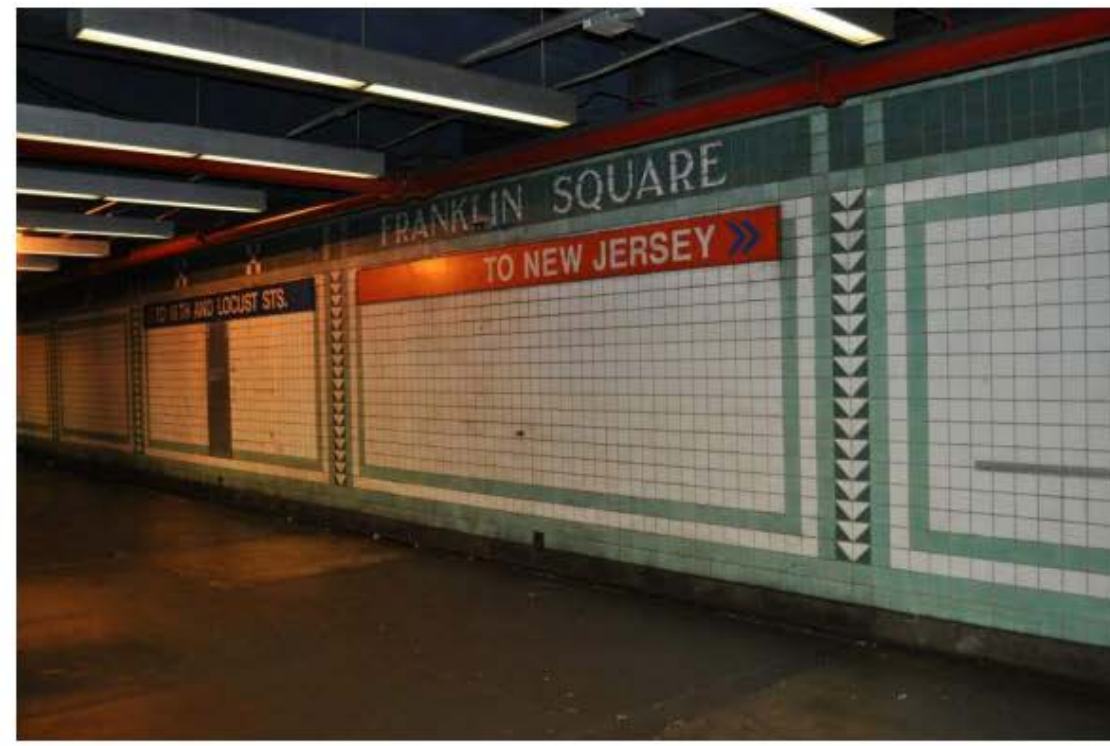
EXISTING CONCOURSE TILING
