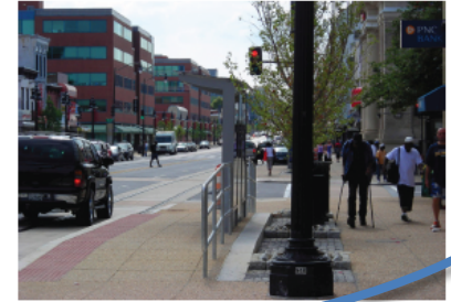
Figure 55 | Curb extension, DC Streetcar Source: BeyondDC via Flickr (CC BY-NC-ND 2.0)
