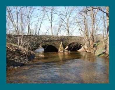
Substantial cracking, missing mortar and bulging spandrel walls
