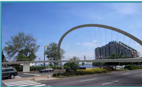
South Street Pedestrian Bridge
