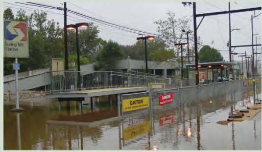
RAILROAD EMBANKMENT AND SLOPE STABILIZATION ($18.7 M)
