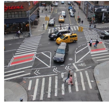
Offset Crossing Pilot treatment, not in widespread use
