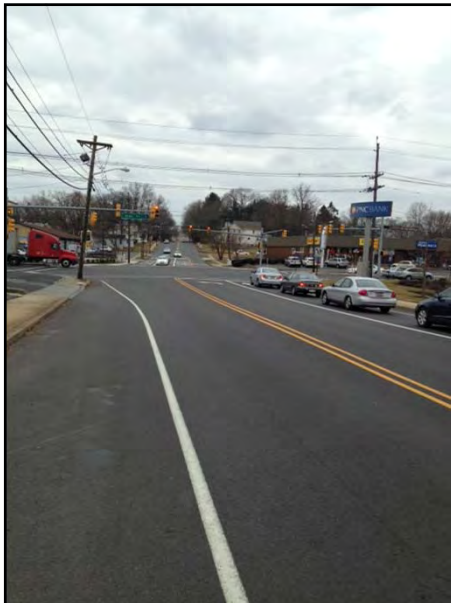
Parkside Ave – Looking South
