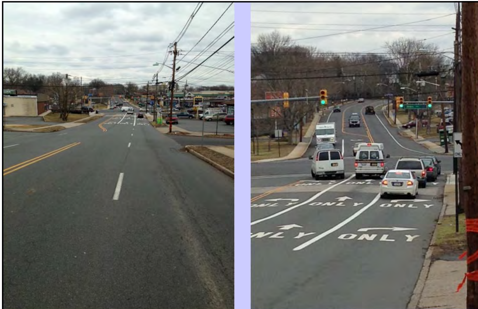
Parkside Ave – Looking North
