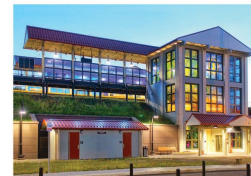
The Pennsylvanian Transit Center, a new station along New Jersey Transit Corporation's NJ TRANSIT Blue Line in New Jersey, completed construction in 2023. Photo Source: Courtesy of NJ TRANSIT
