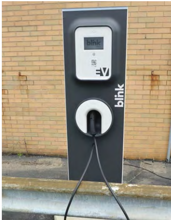
Electric Vehicle Charging Stations
