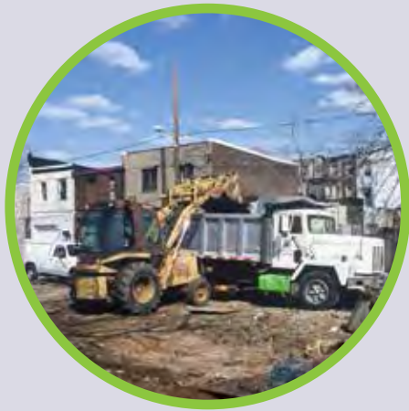
Major trash, debris, and weed removal
