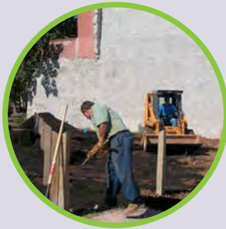
Site grading and seeding
