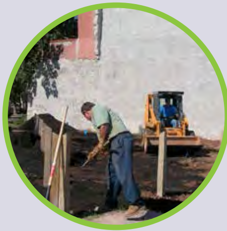
Site grading and seeding
