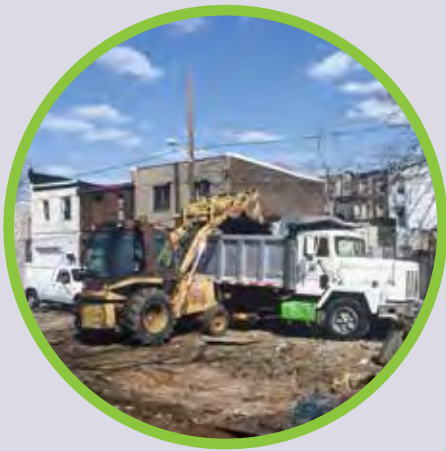
Major trash, debris, and weed removal
