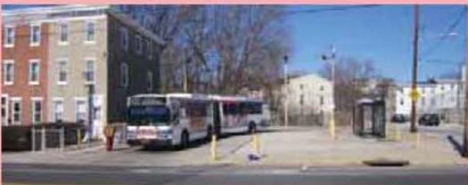
35th and Allegheny Streets Bus Facility (Planned)
