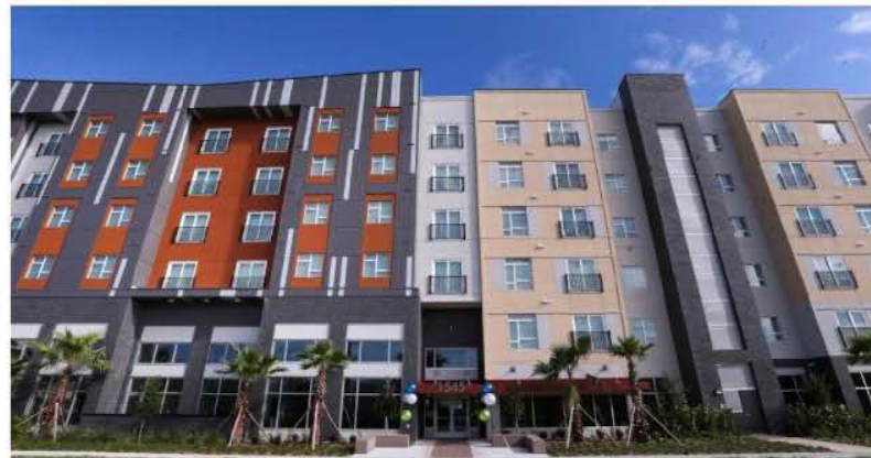
The Renaissance at West River in Tampa, Fla., is the first apartment complex to be completed in the West River urban renewal project. The six-story, 160-unit complex is a part of Tampa's commitment to provide 10,000 affordable housing units by 2027. (Dirk Shadd/Tampa Bay Times/TNS)
