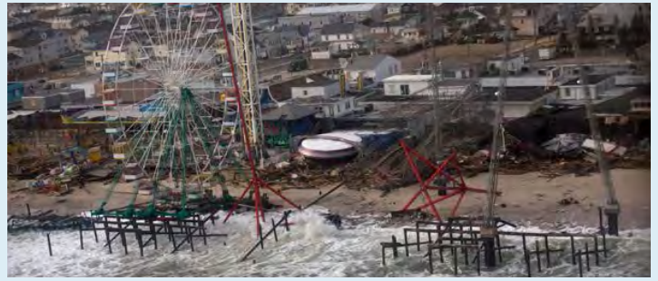
Seaside Heights in the aftermath of Hurricane Sandy. Official White House photo by Sonya N. Herbert.
