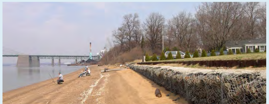
This beach in Pennsville along the Delaware River could be lost as sea level rises, if the shore erodes up to the shore protection wall to the right. © James G. Titus; used by permission.
