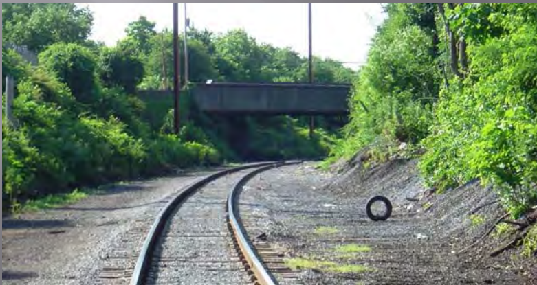
York Road (MP 8.07) Looking west
