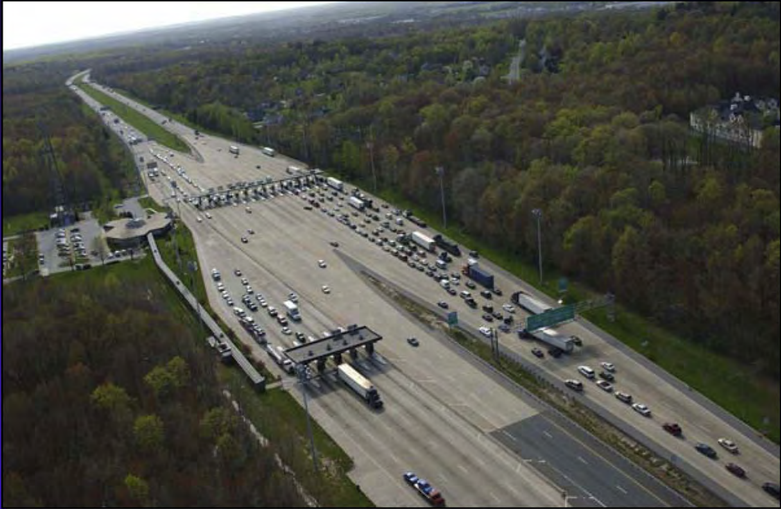
I-95 Newark Toll Plaza
