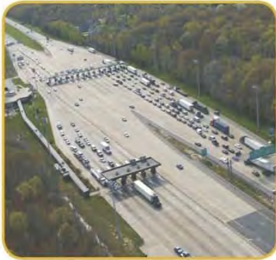
The existing Newark I-95 Toll Plaza experiences back-ups and delays.
